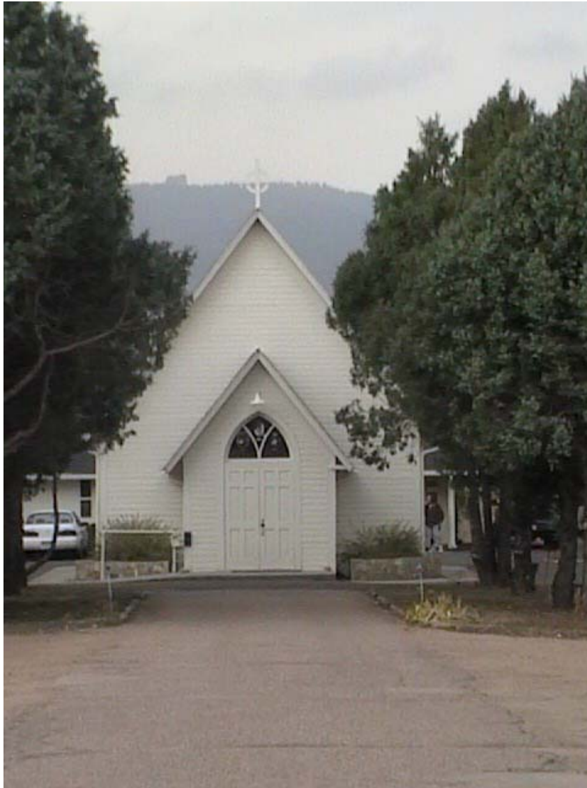
St. Philip Episcopal Church (1 st Church built in Douglas County)
